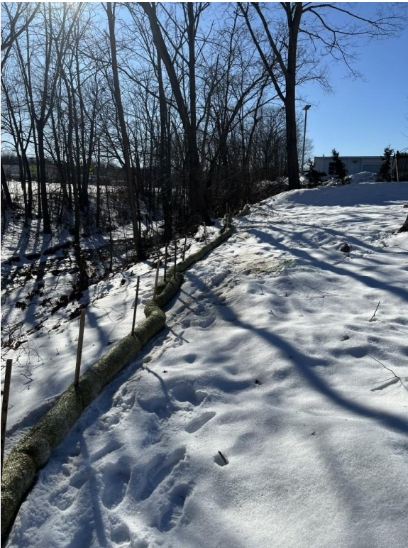
Photo 11. Silt sock erosion control measures installed at the top of the embankment above Hodgson Brook. Photo provided by the property owner.
